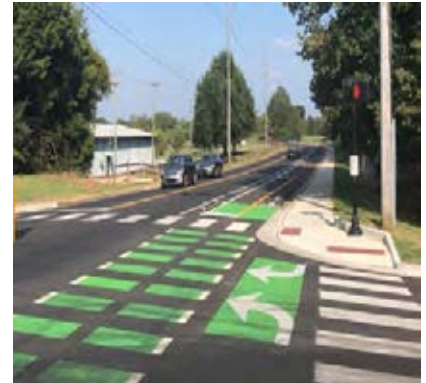
Pedestrian and Bicycle Crossing, MSU South Entrance
